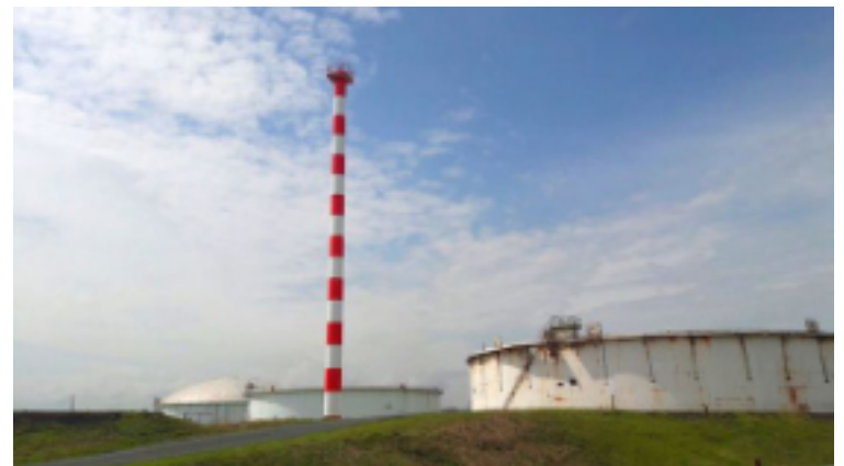
The ALT 7 modular beacon of galvanised and painted steel by Almarin, manufactured in Portugal, supplied to the Panama Maritime Authority.
