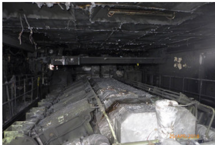
Fire damage to upper engine room (looking forward)
